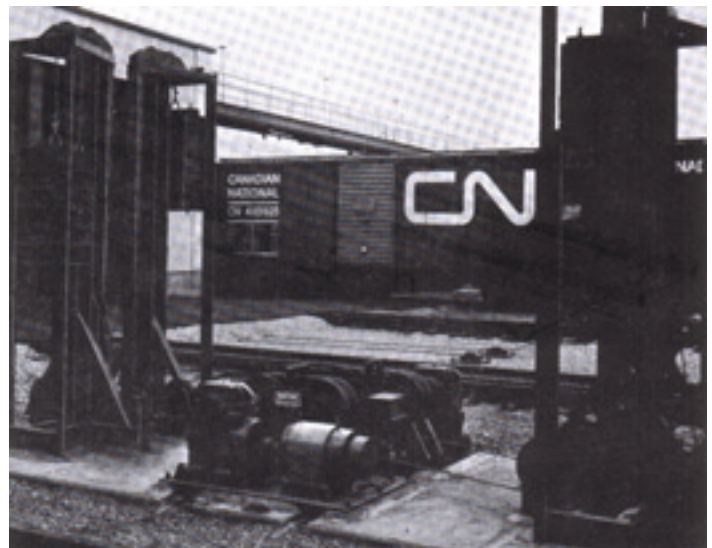
ROBOT arms ride in covered track between rails, rise to contact axle, side frame or coupler, according to design.
